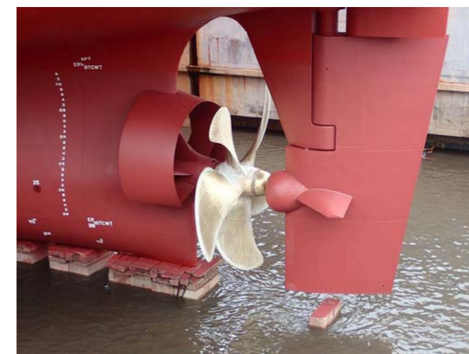
Installation of propeller duct on M/T Hampshire
